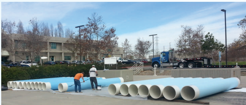
Because these pipes will be outside and exposed to the sun, a special paint is used to protect the pipes from the sun's ultraviolet rays.
