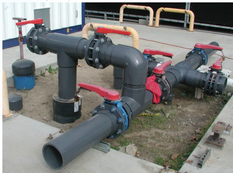
The recycled water produced at the North City Water Reclamation Plant will be directed to ozonation and BAC filters prior to the AWP Facility’s 3-step water purification process. Additional piping was installed to direct the recycled water to the new equipment.
